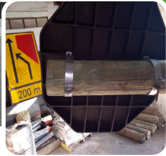
Figure 15: Used sanky clamp system to fix rubber sign to timber post.
