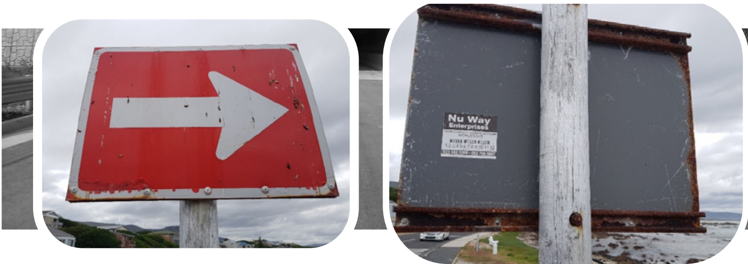
Figure 4: Condition of galvanized signs exposed to coastal conditions.
