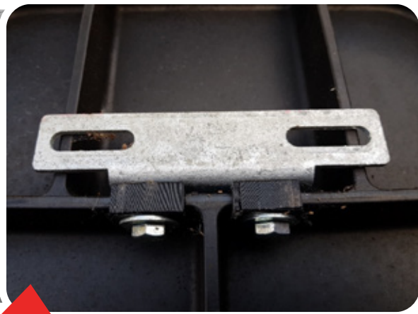
Figure 14: Photo of the fixed bracket
